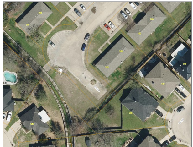
FIGURE 2. 2023 AERIAL IMAGE SHOWING THE IMPROVED RIGHT-OF-WAY TERMINATING INTO THE REAR YARD OF 153 SOUTHWOOD DRIVE
